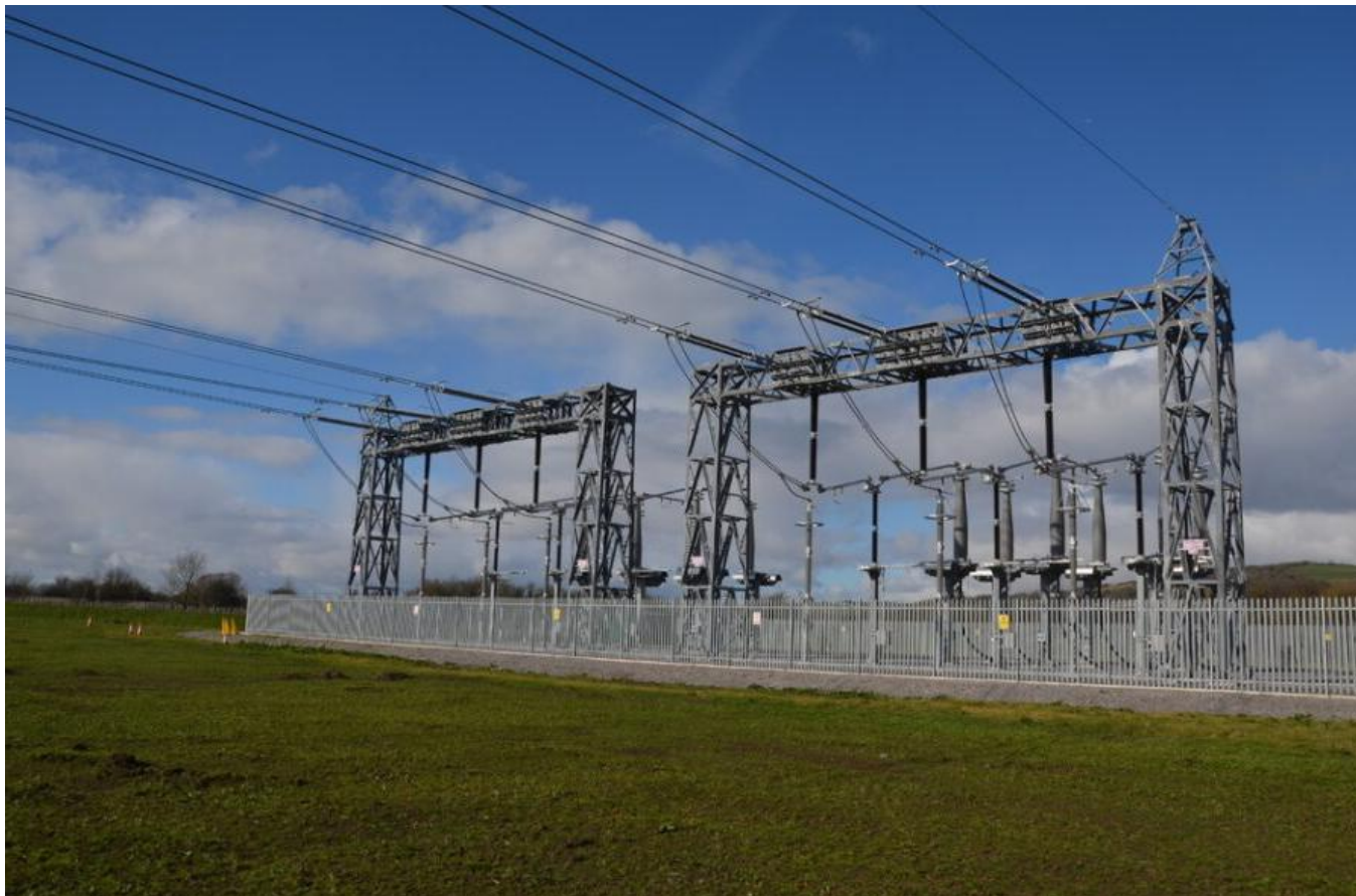
Image 3.9 Existing CSE compound with gantries (Source: ES Chapter 4: Project Description (Revision B))
